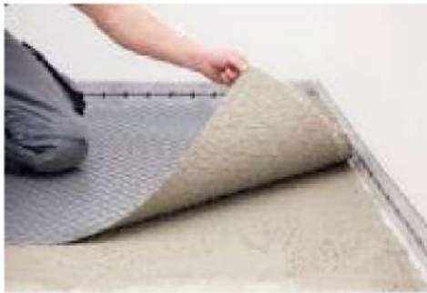
Lay the Decoupling Pad
