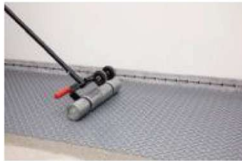
Smooth the Decoupling Pad
